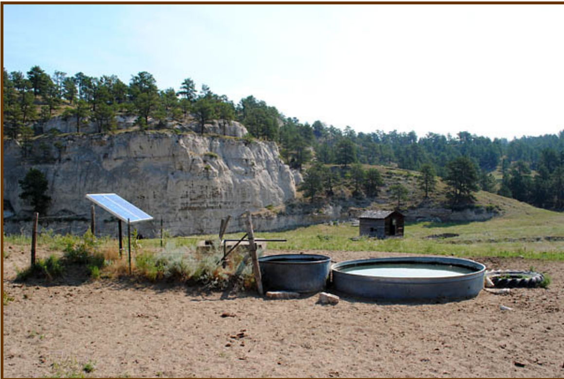
Within the past couple of years, a solar well has been placed on the ranch to enhance the water supply.
